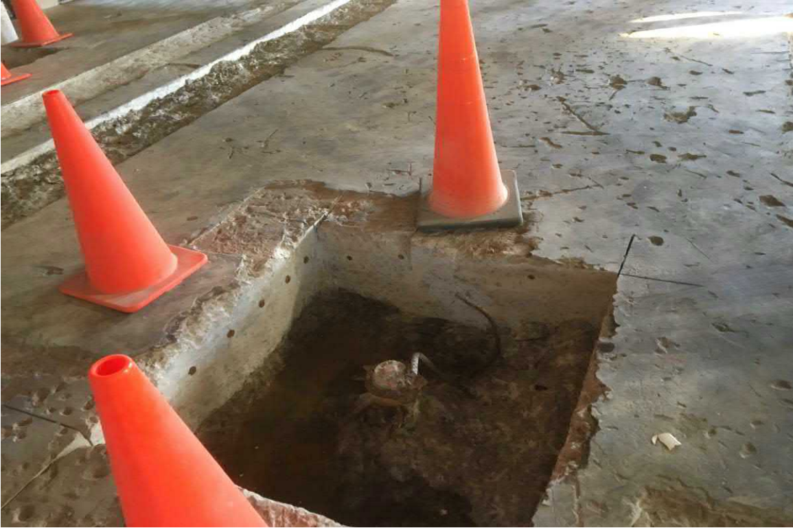
View of Concrete Slab Thickness / Industrial Areas
