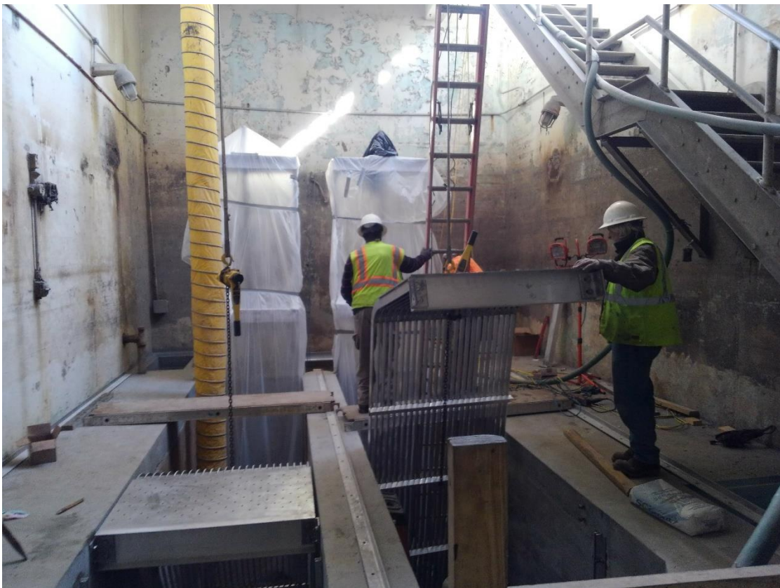
Noisette PS Rehabilitation: new bar screens being installed into the channels
